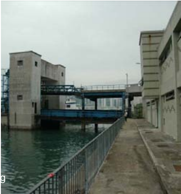
Abandoned two-level vehicular ferry pier.
