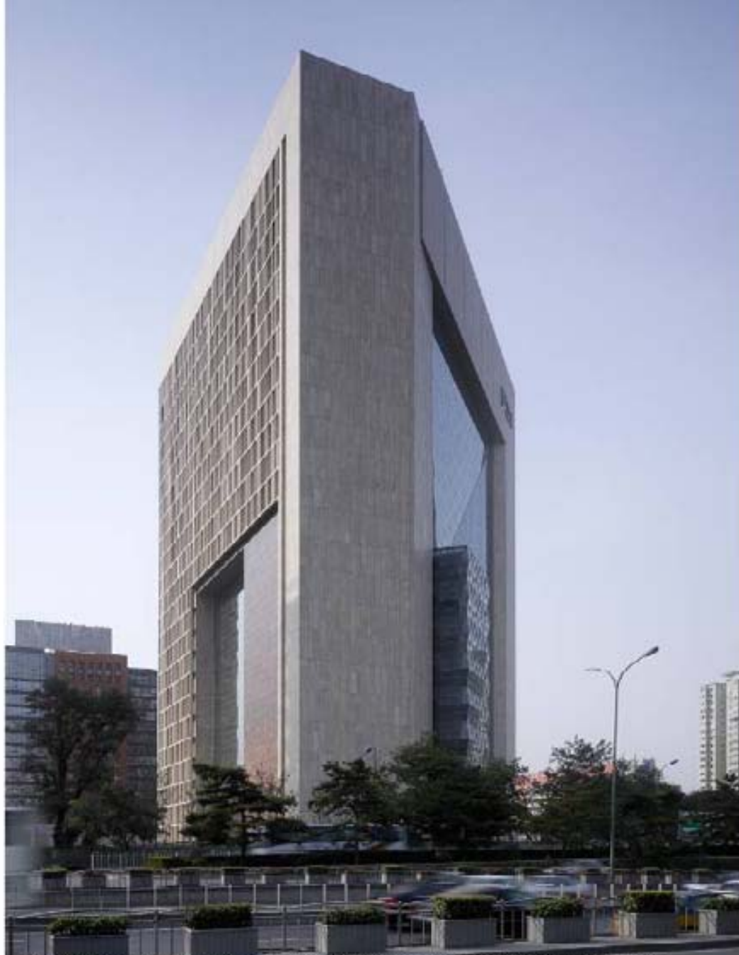
The triangular shape minimizes the perimeter surface exposed to the elements, while the interior atrium draws daylight into office areas.
