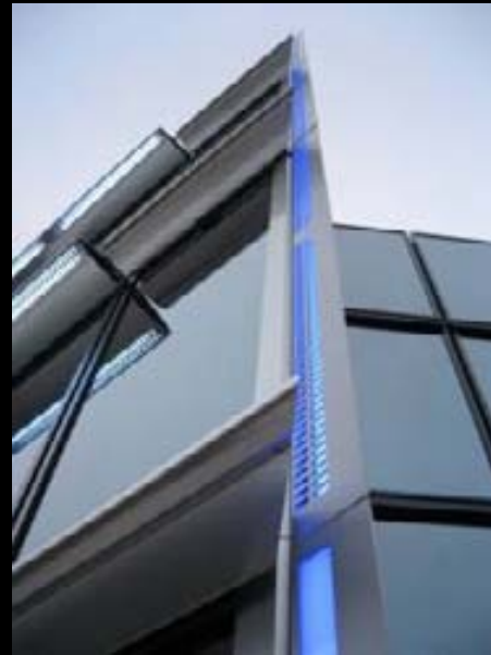
Exterior LED Lighting
